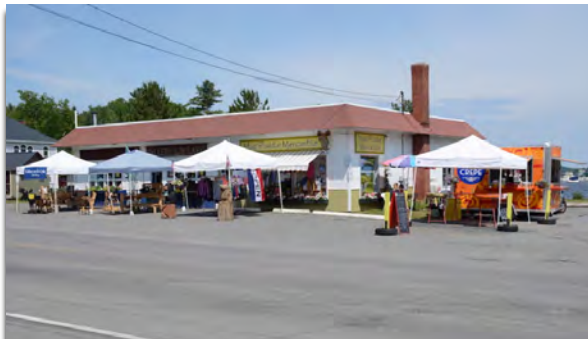
Underutilized pavement with no defined pedestrian sidewalk or parking areas.
