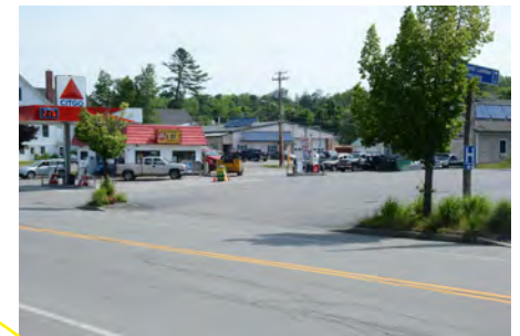
Underutilized pavement, wide curb cuts, and minimal landscaping discourage pedestrians from walking along road.
