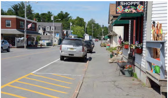
Cross walks and parking at intersection not well defined
