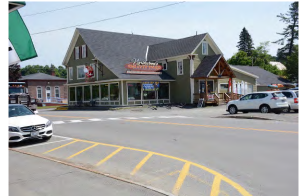
View looking northeast at Moosehead Lake Road. On-street parking and cross walks need to be redefined. Conflict at intersection with left turning traffic and through traffic heading north.
