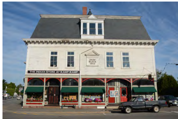
The Shaw Block preserves the Greenville's architectural heritage as one of the oldest buildings in downtown
