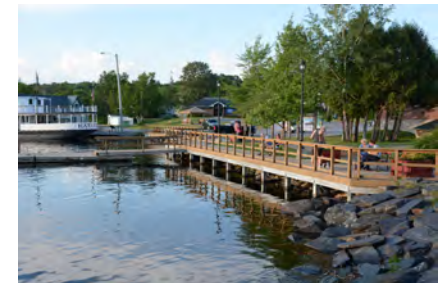
Boardwalk and interpretive signage
